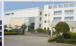
佛山·禅城工厂 Foshan Chancheng Production Base
